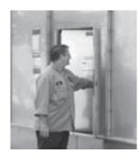
the access doors are 48" high. Small access doors are prohibitive and discourage maintenance, which in turn can impact your operation. Specifying the size of the door will cause some bidders to take exception, alerting you to a potential maintenance headache. Two doors are standard on all Series Quiet Class towers—one in each endwall.
